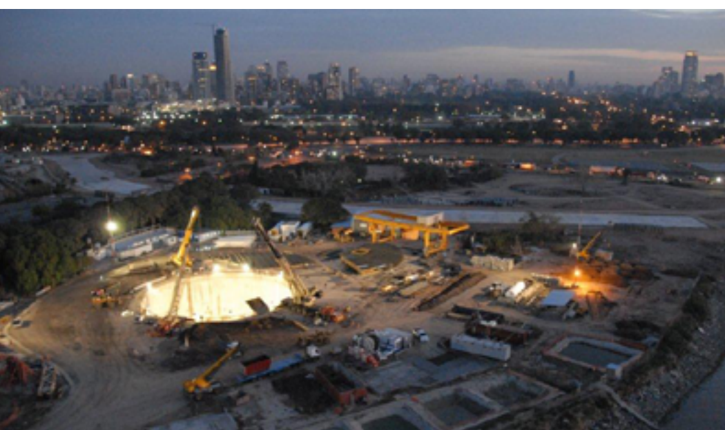
Ghella's Maldonado construction site Buenos Aires (Argentina).
